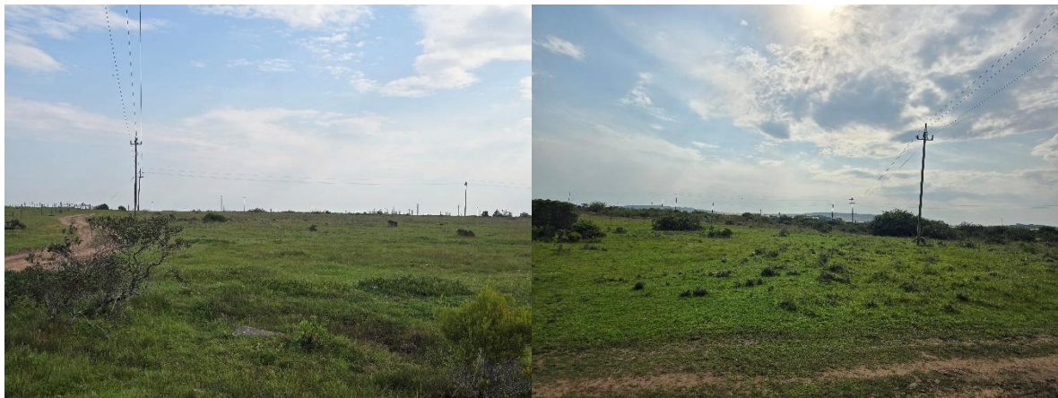
Figure 53: Existing powerlines within the Project site
